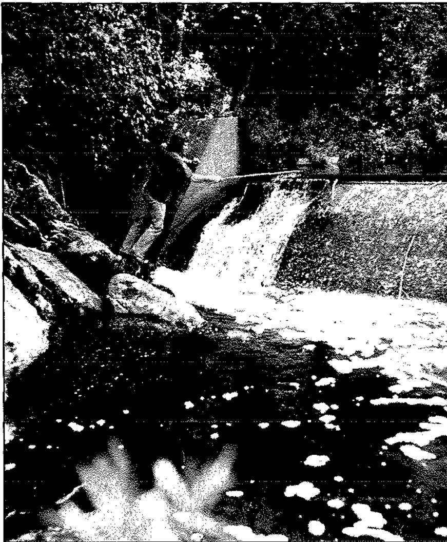
A research worker is seen removing an obstruction at a weir on a river in the Wilderness catchment area
