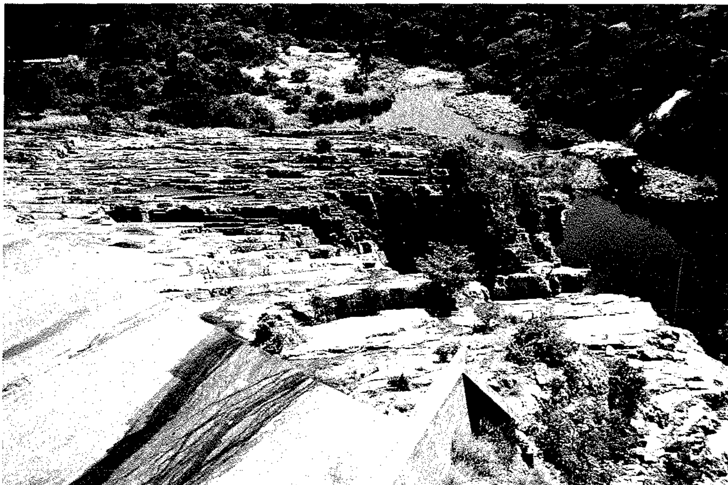
Area downstream of the concrete canal at the Hartbeespoort Dam
