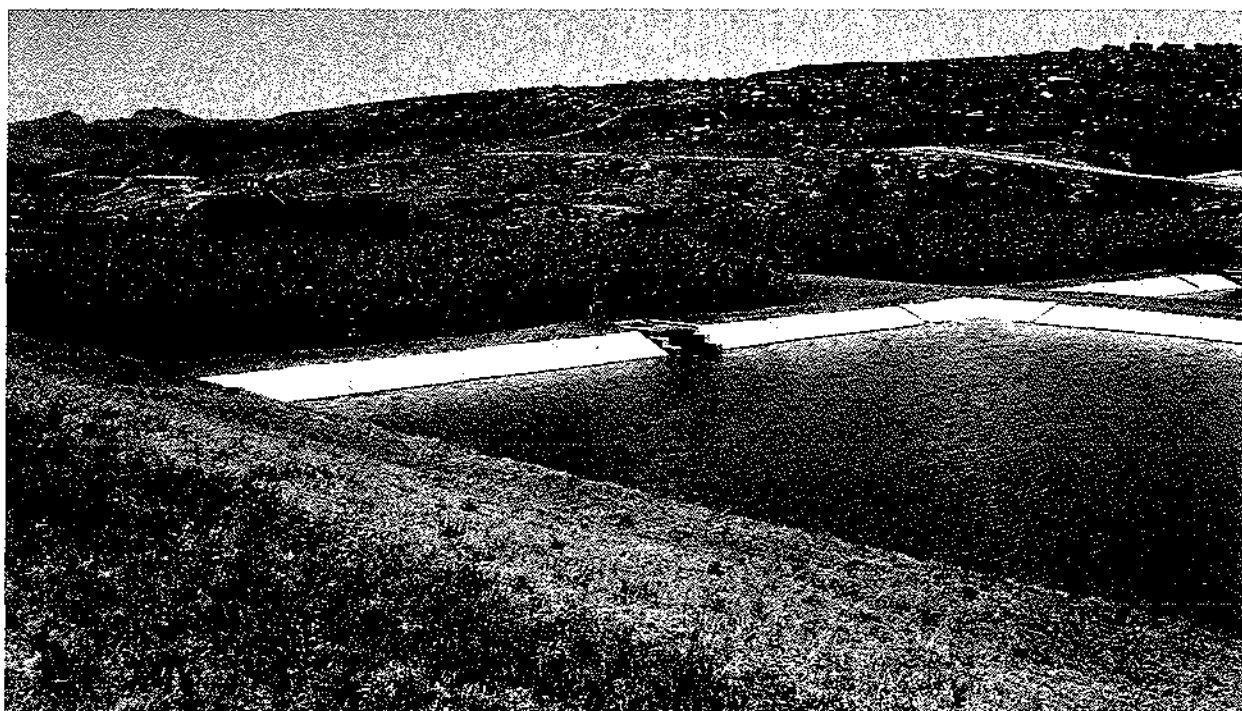
A full-scale constructed reedbed for waste-water treatment in Qua-Qua
