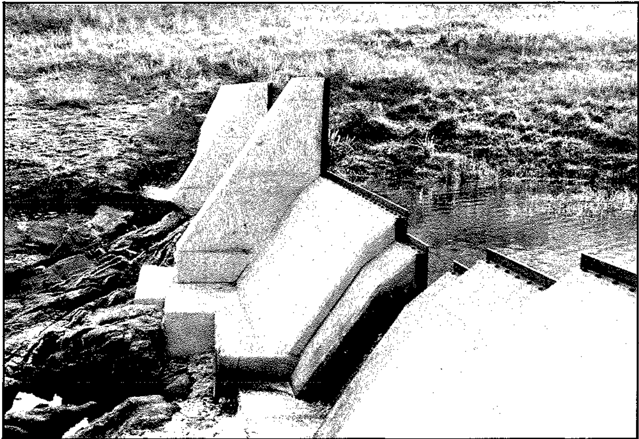
A weir in the Mtunzini catchment being used for studying runoff in small catchments.
